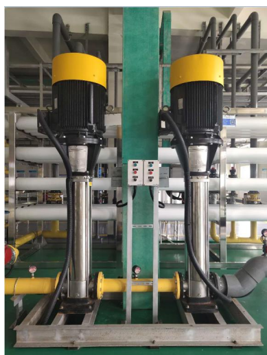
减振基座和软连接
